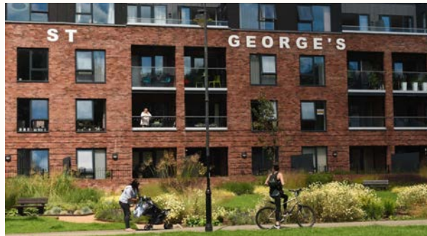
St Georges Works, Trowbridge
