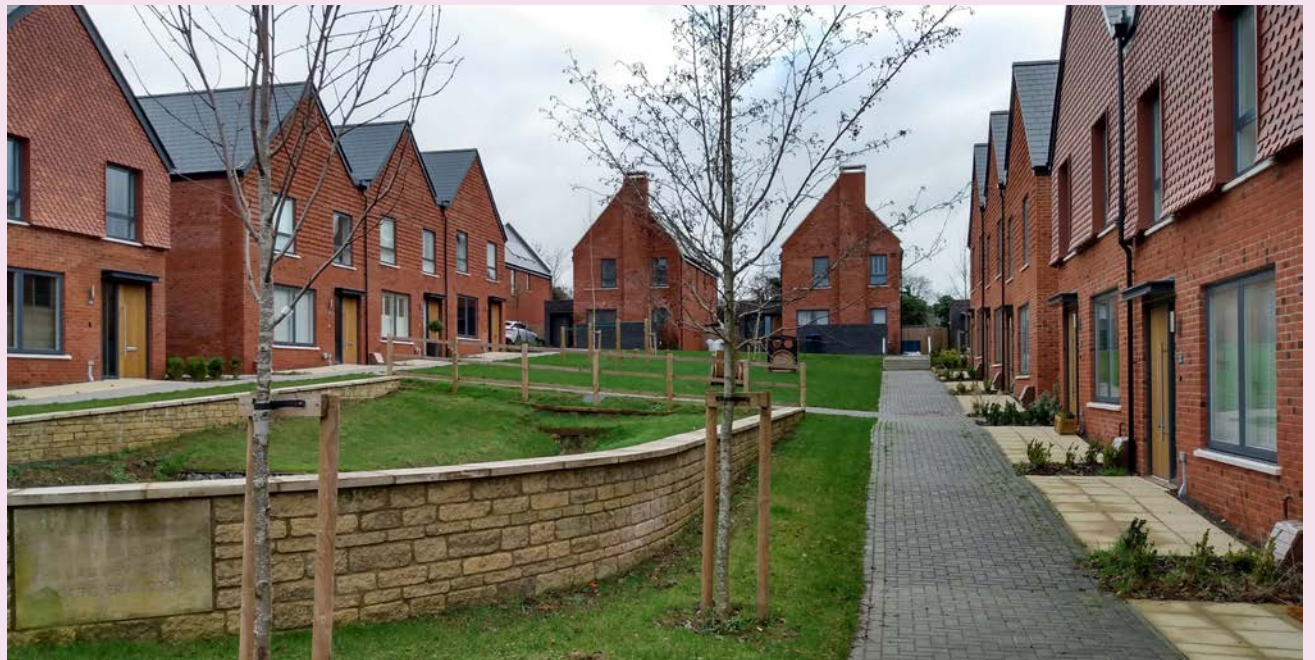
Distinctive gables, tile hanging and chimney stacks, Former Westbury Hospital.
