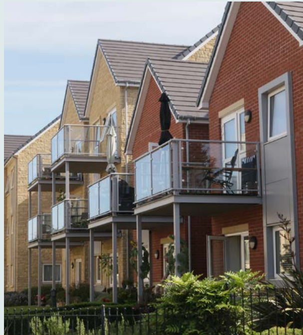
Supported living, within walking distance of town centres, Waterford Place, Chippenham
